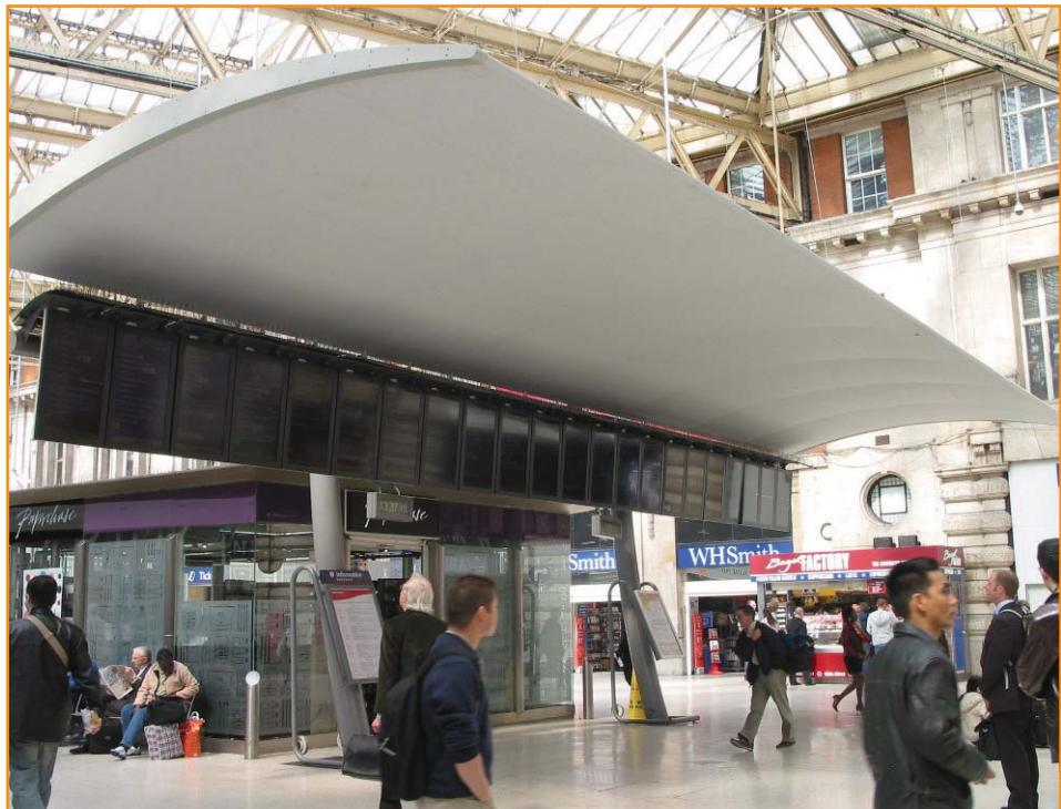
*This picture shows the old plasma screen installation at Waterloo station before it was ripped out and replaced with LEDs. The glare off the front face of the boxes is very clear, as is the lack of brightness of the plasma panel itself.*
