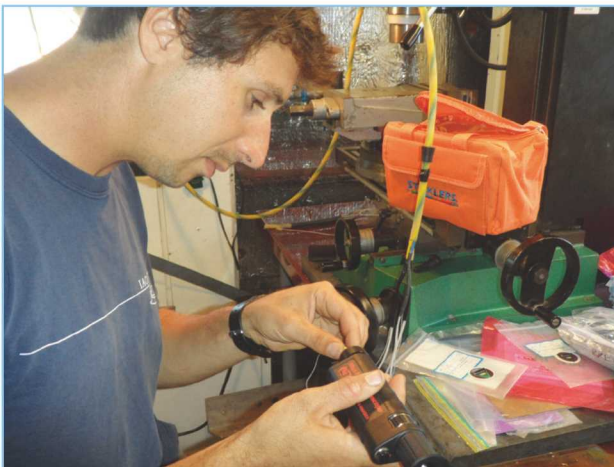
Figure 5: An essential element in the cleaning process is to inspect every end-face properly after cleaning. Here the operator has installed a new connector on the fibre optic cable and is inspecting with a simple, handheld scope. Every technician who touches any fibre must be equipped with at least a low-power inspection scope
