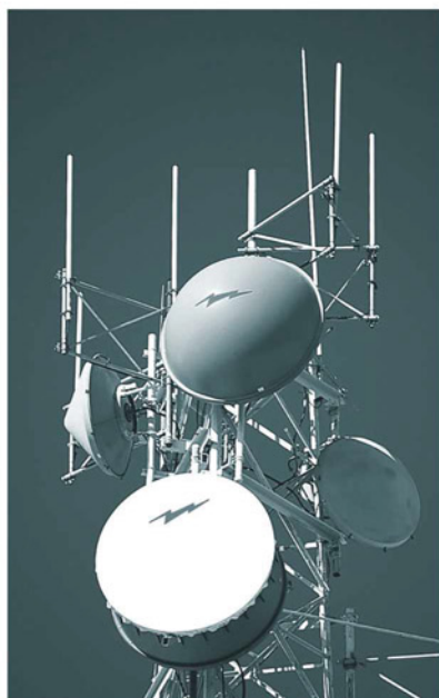
Microwave systems are the most common form of backhaul at wireless cell sites
